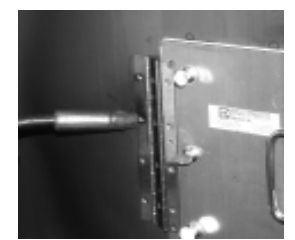
8. For hinged door, position hinge on duct wall and plug weld.
