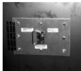
7. Install thumbscrews with washers.
