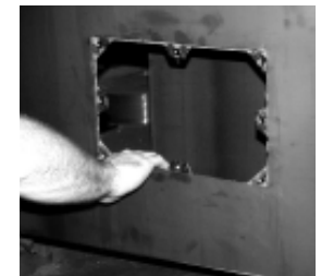
4. Center the frame around the opening.
